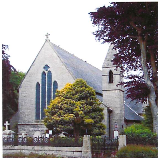
St John the Evangelist Episcopal Church built 1871 of granite from the local quarries
